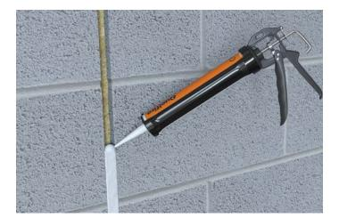
QuelStop CE Marked Intumescent Acrylic Sealant forms part of a lifesaving system designed to prevent the spread of fire through compartment walls and floors, it is therefore essential that the product is installed in a responsible and workmanlike manner with life safety in mind.
