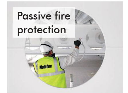
Intumescent Coatings, Fire Stopping
