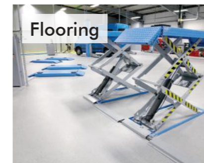
Seamless Resin Flooring, Subfloor Preparation, Car Parking Structures
