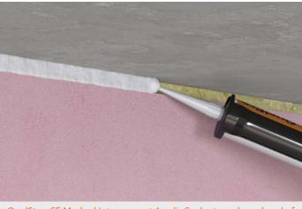
QuelStop CE Marked Intumescent Acrylic Sealant used as a head of wall linear joint seal
